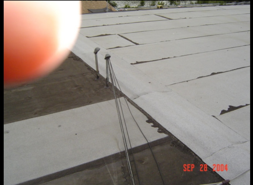
Leaking Control Joint
