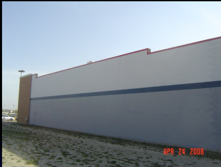
Painted Concrete Block Wall
